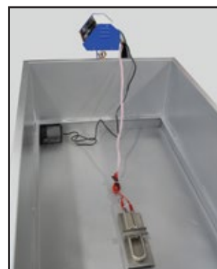
Internal Tank View
